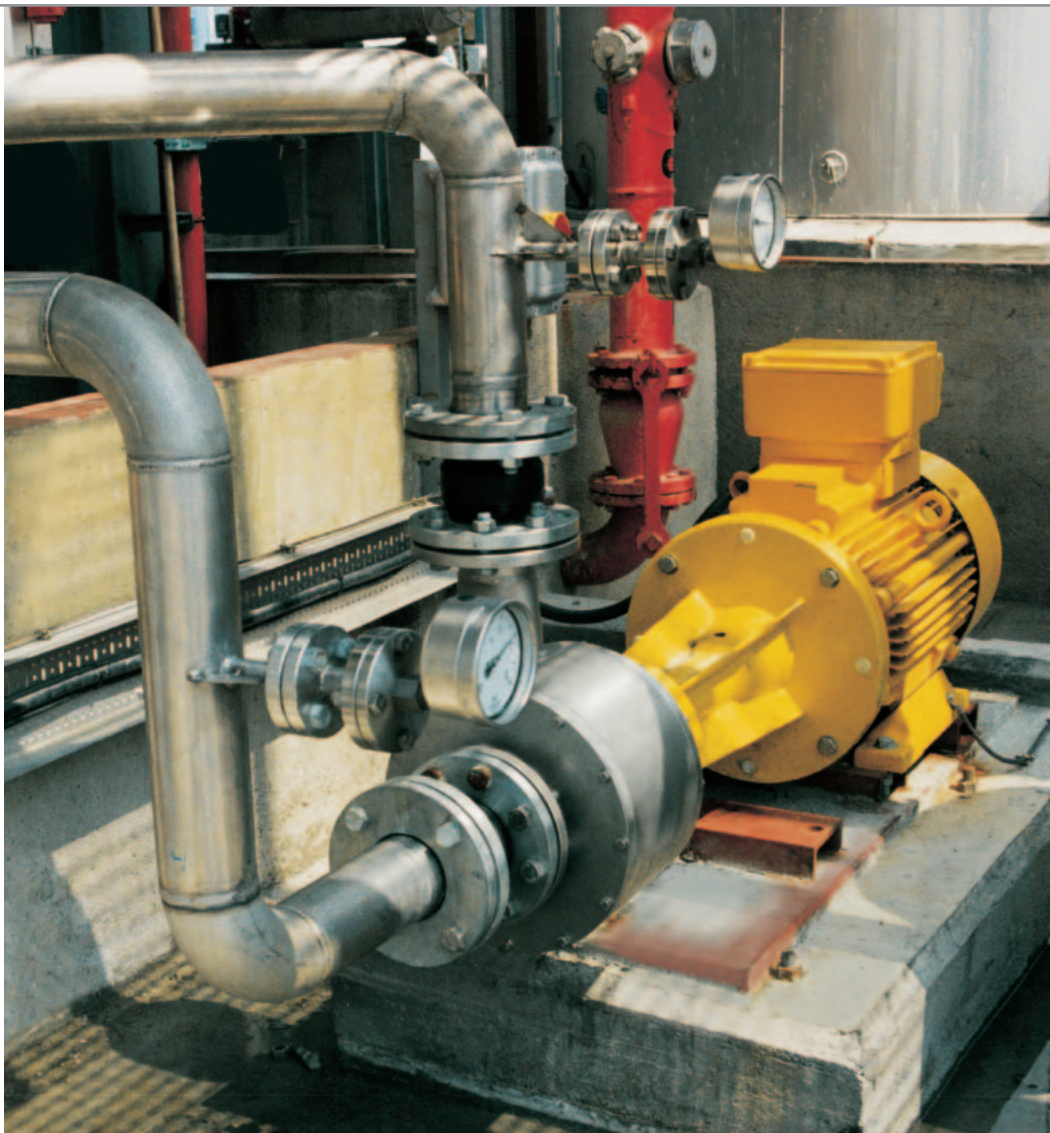
YTRON-Z in the Chemical Industry Application: Homogenising of Liquid Detergent Emulsions
